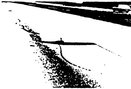
Fig. 3.2.4.2 — Meandering crack
